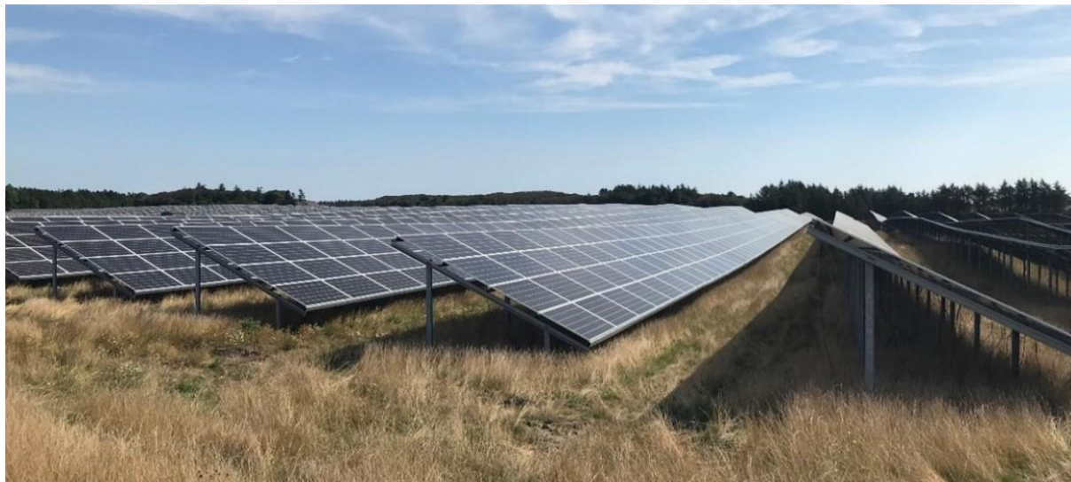
Figur 5. Fast monterade solpaneler, s.k. "fixed tilt".
