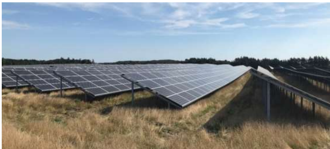
Figur 4. Fast monterade solpaneler, sk. "fixed tilt".
